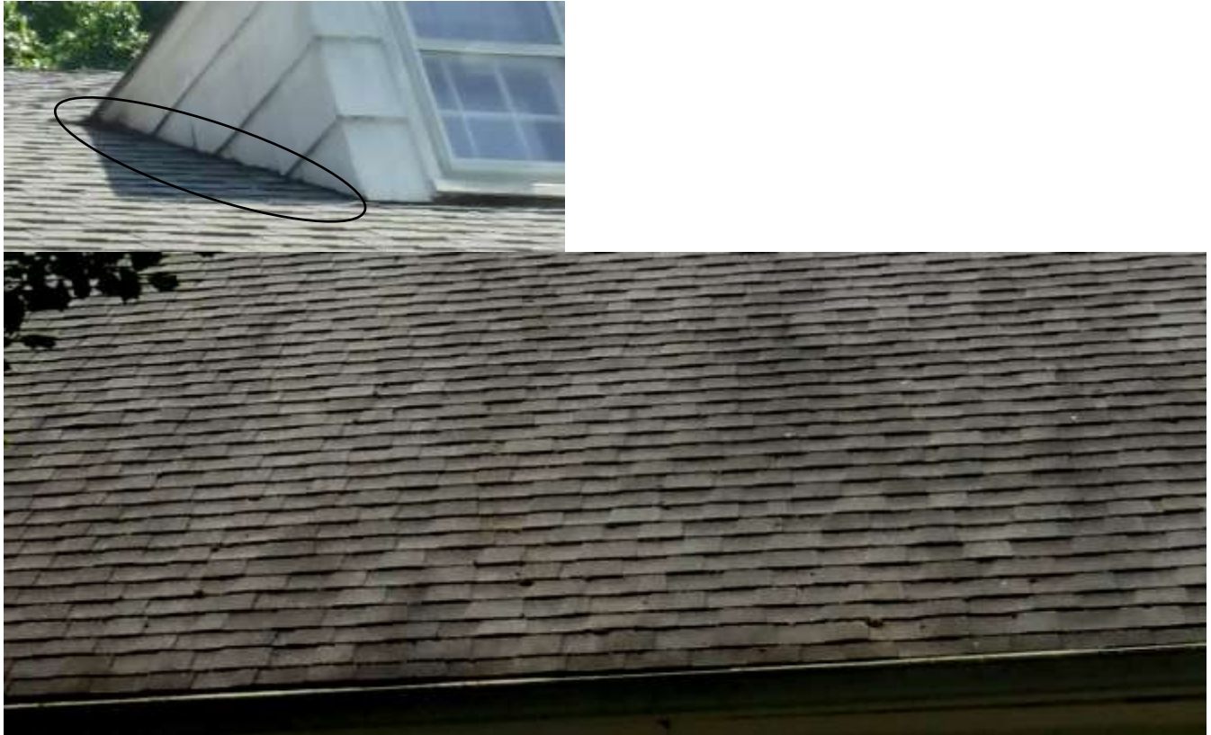
Figure 1 Example of heavy moss build, granular loss, curling, staining, brittle, etc.
