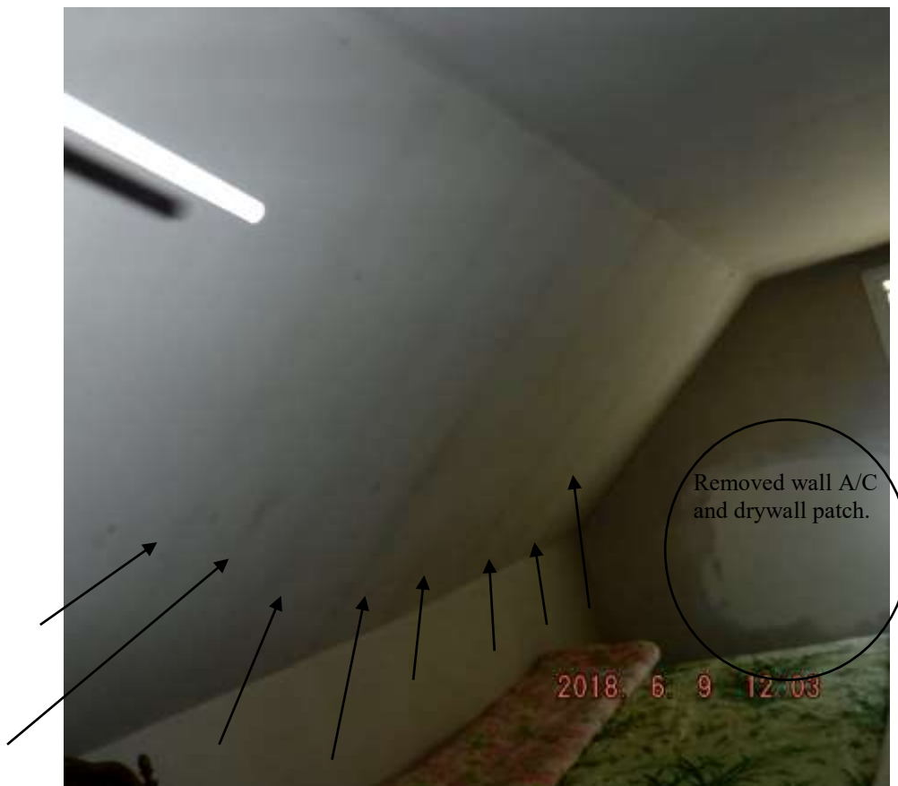
Figure 10 Example of "Ghosting or thermal bridging" in the home. Recommend an insulation & ventilation contractor evaluate home and advise on a proper mix of both. See roofing & attic section comments.
