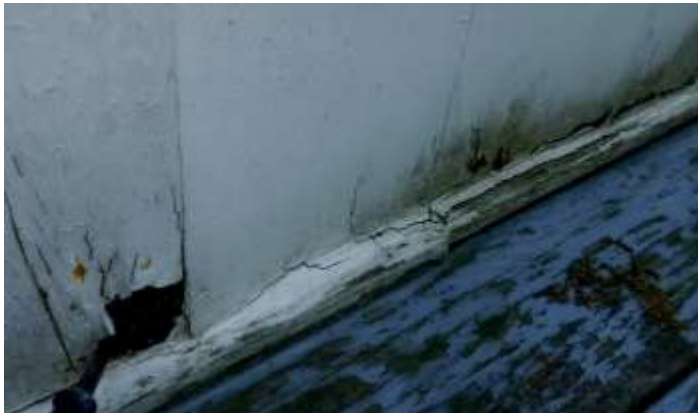
Figure 4 Example of carpenter bee damage. See separate NPMA-33 Wood destroying insect report.
