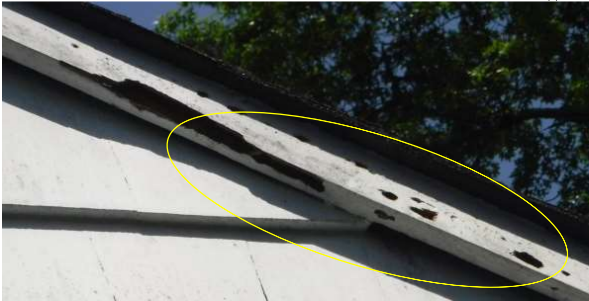
Figure 4 Example of carpenter bee damage. See separate NPMA-33 Wood destroying insect report.
