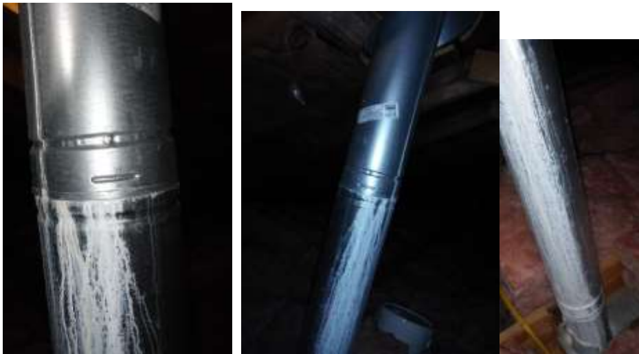
Figure 4 Chimney was dented/crimped/gaps, white condensate residue (joints/connections); improper installation/drafting concerns/safety concerns.
