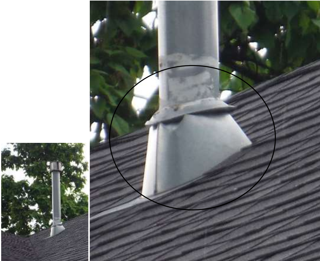
Figure 4 Chimney was dented/crimped/gaps, white condensate residue (joints/connections); improper installation/drafting concerns/safety concerns.
