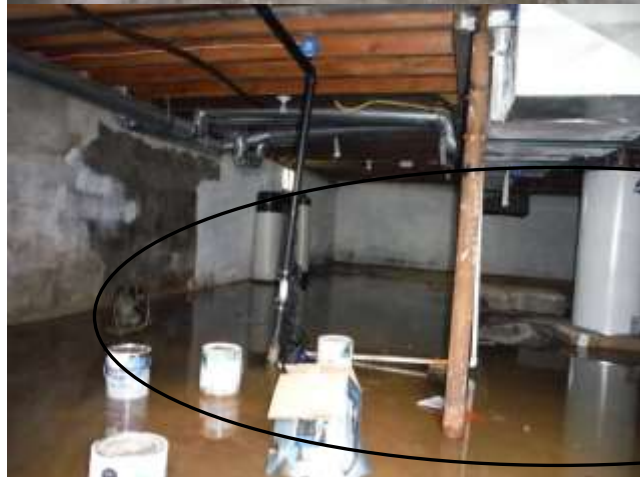
Figure 7 Left addition crawl space had duct work & insulation along with water (2" plus) on basement floor (camera zoom shot); inaccessible.
