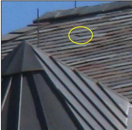
Figure 39 A , B & C Examples of broken or chipped slate.
