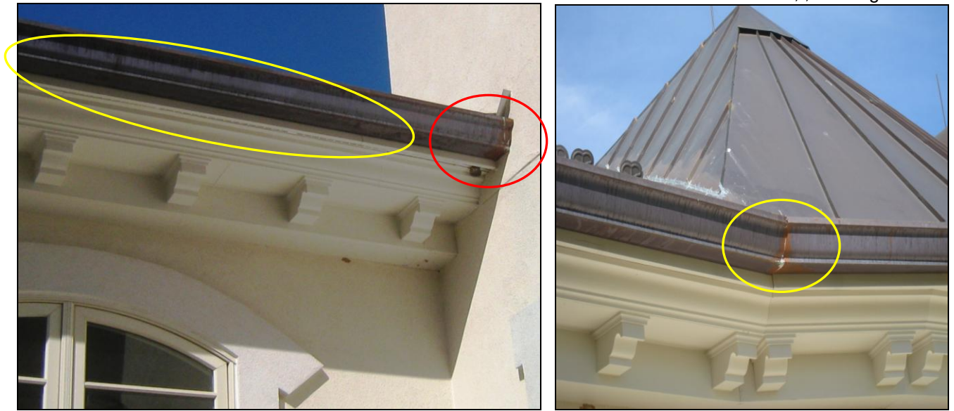
Figure 15 A, B, C & D Indication of leaking gutters and spillage marks. Ruts in soil below.
