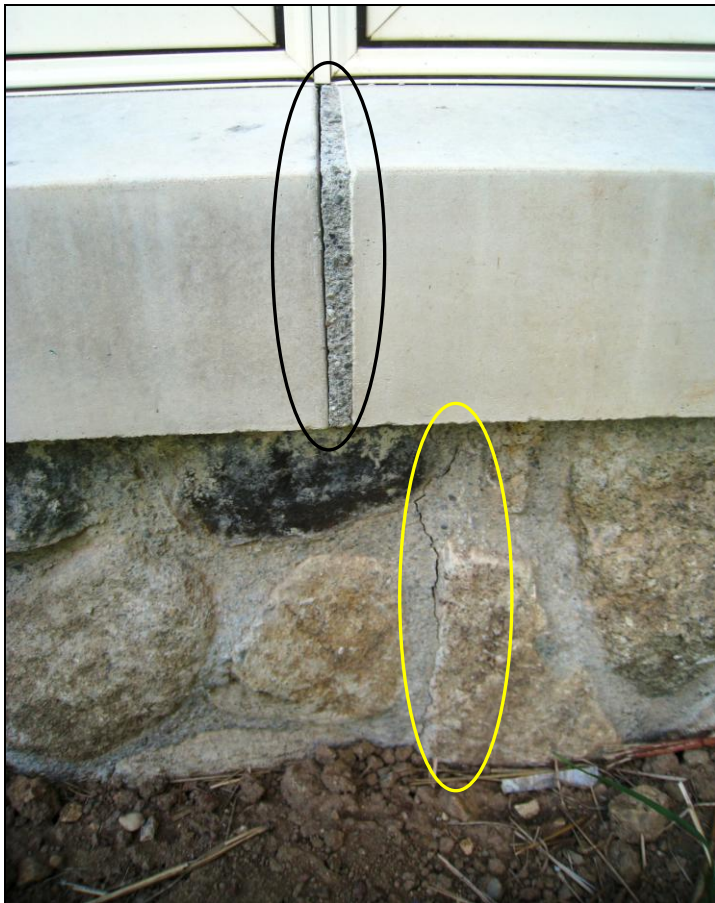
Figure 21 Several vertical cracks all around outcrop main kitchen area. Recommend evaluation by Structural Engineer; structural concern.
