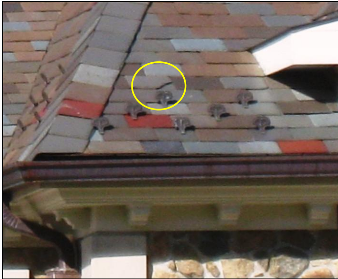
Figure 11 A & B Example of broken slate shingles
