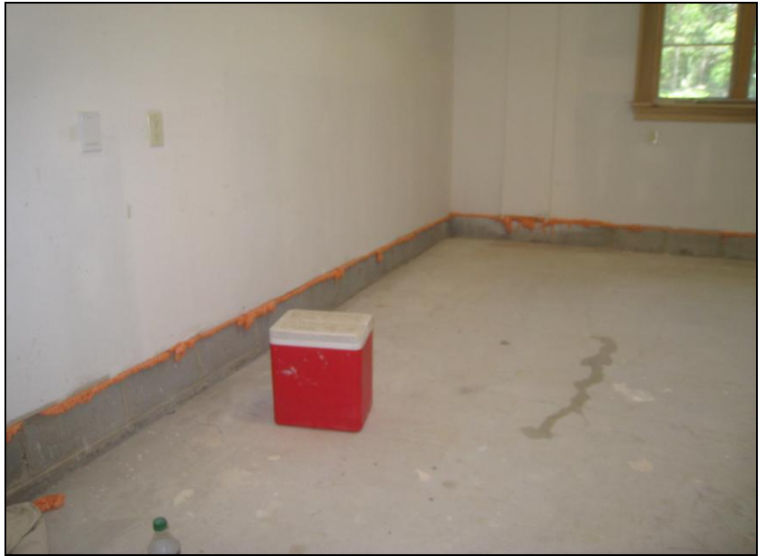
Figure 50 Loose wires by garage doors; further evaluate. Expansion foam everywhere; not recommended.
