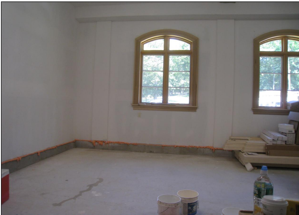
Figure 50 Loose wires by garage doors; further evaluate. Expansion foam everywhere; not recommended.
