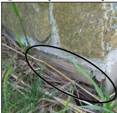
Figure 47 Wood forms left under stone and in contact with soil(siding & retaining walls)
