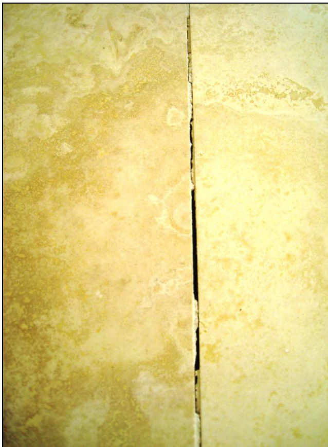
Figure 51 Numerous cracks on tiled flooring in living room; have evaluated and corrected.
