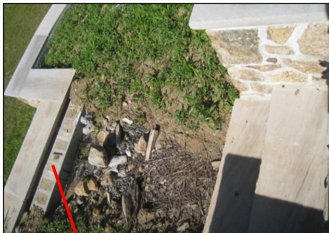
Figure 1 A & B Missing walk between retaining walls; fall hazard.
