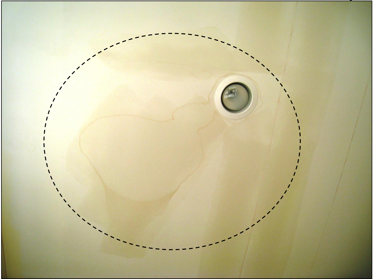
Figure 52 Water stains; indication of leaking above. See roofing section.
