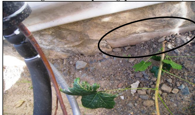
Figure 47 Wood forms left under stone and in contact with soil(siding & retaining walls)
