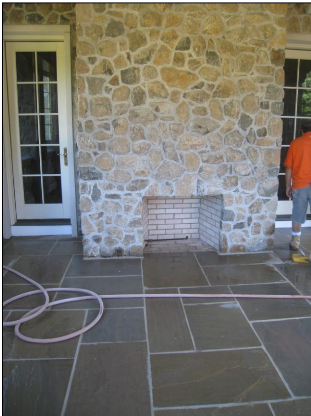
Figure 35 Slate/mortar repairs being made.
