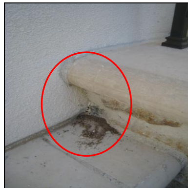
Figure 16 Gaps in caulking/mortar and ant hills. Gaps under rear door.
