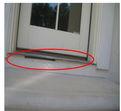
Figure 43 Gaps in caulking/mortar and ant hills. Gaps under rear door.
