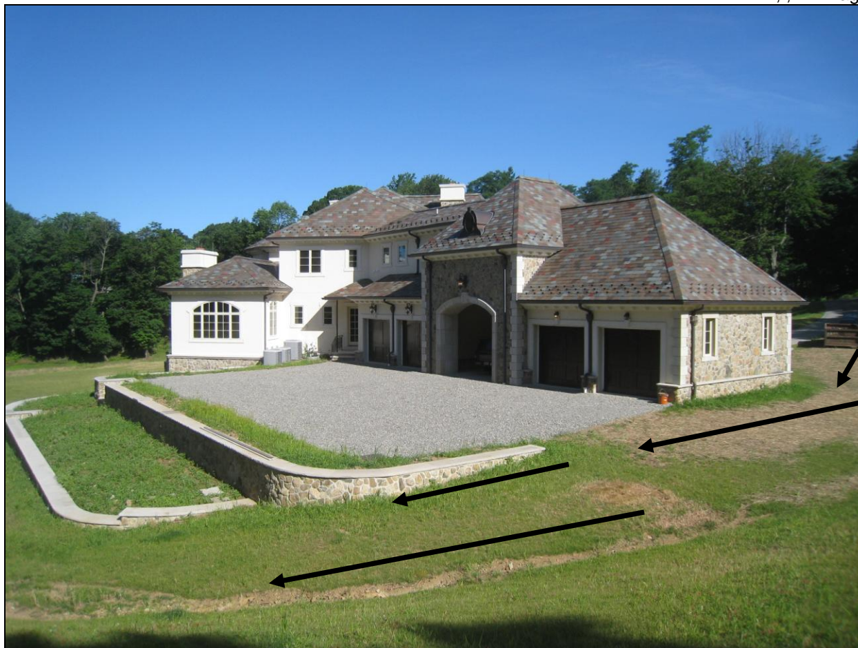
Figure 4 Deep ruts where water washing away soil from front driveway to side/rear property; drainage concerns.
