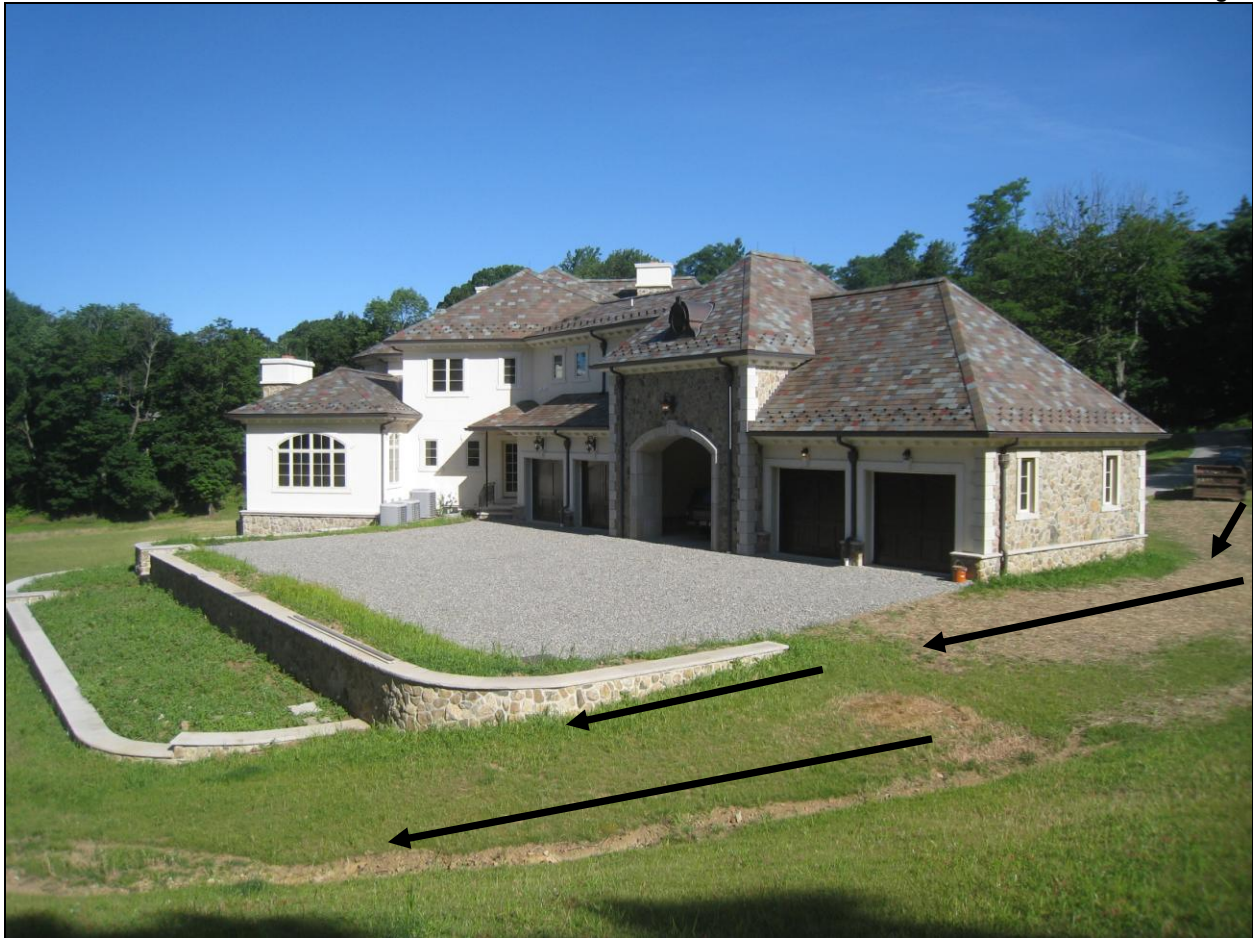
Figure 31 Deep ruts where water washing away soil from front driveway to side/rear property; drainage concerns.
