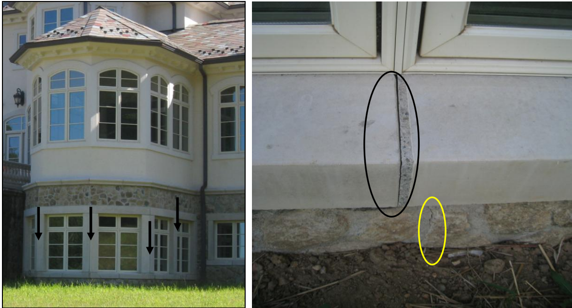
Figure 48 Several vertical cracks all around outcrop main kitchen area. Recommend evaluation by Structural Engineer; structural concern.
