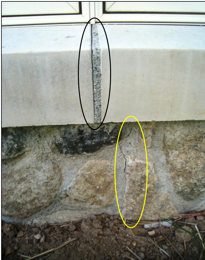
Figure 48 Several vertical cracks all around outcrop main kitchen area. Recommend evaluation by Structural Engineer; structural concern.
