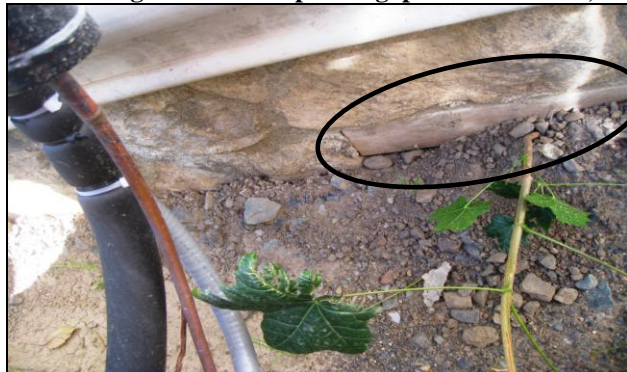
Figure 20 Wood forms left under stone and in contact with soil(siding & retaining walls)
