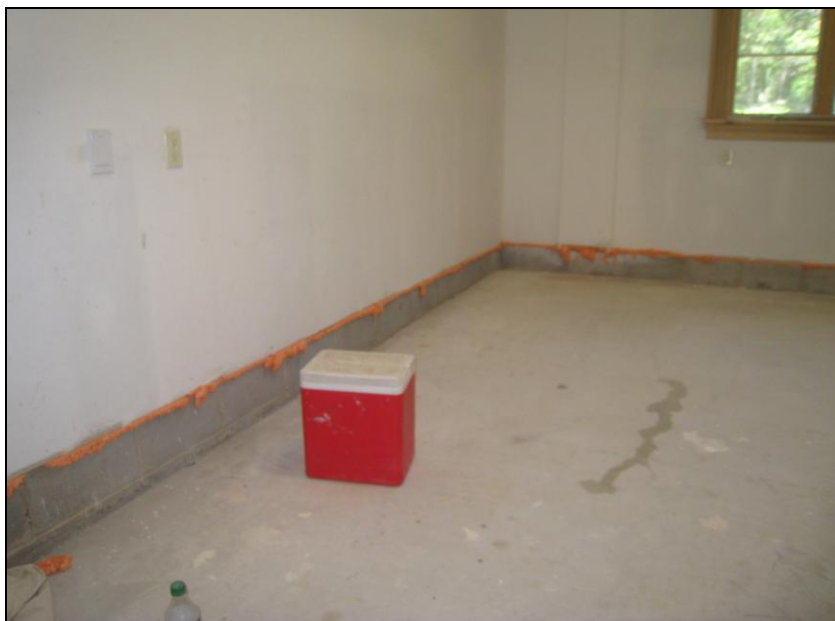
Figure 23 Loose wires by garage doors; further evaluate. Expansion foam everywhere; not recommended.
