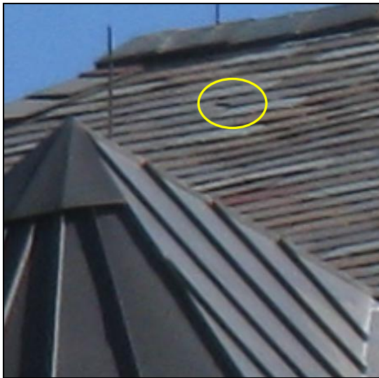
Figure 12 A, B & C Examples of broken or chipped slate.
