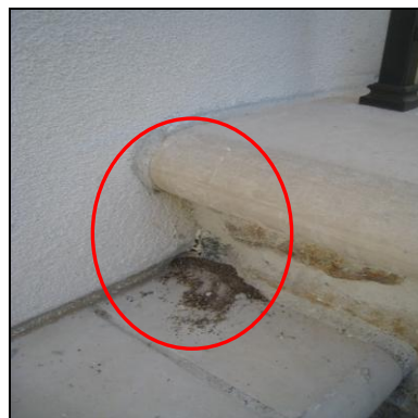
Figure 43 Gaps in caulking/mortar and ant hills. Gaps under rear door.
