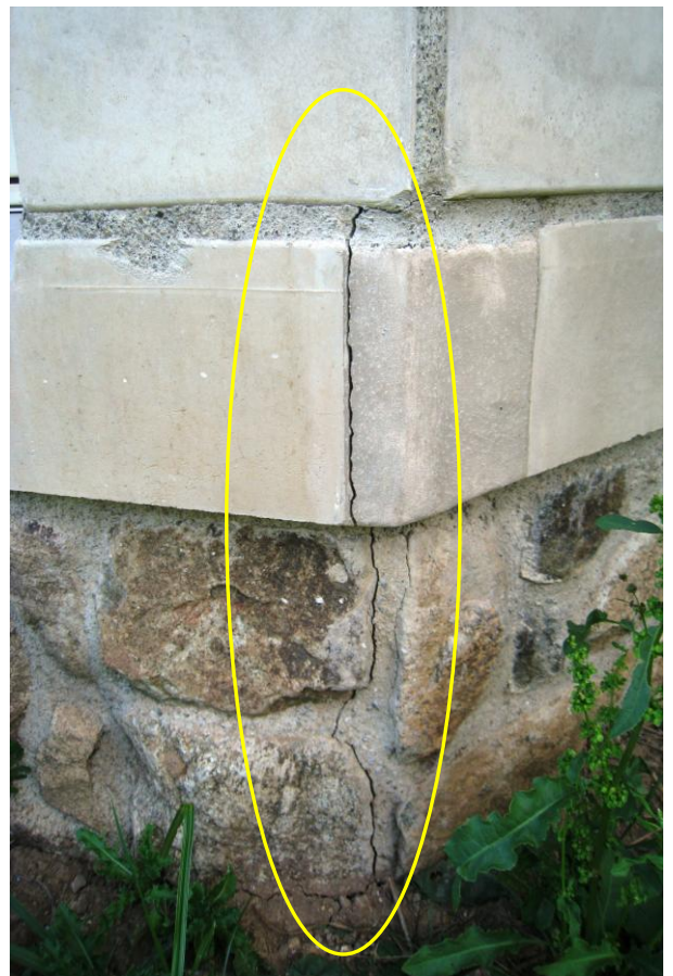
Figure 21 Several vertical cracks all around outcrop main kitchen area. Recommend evaluation by Structural Engineer; structural concern.
