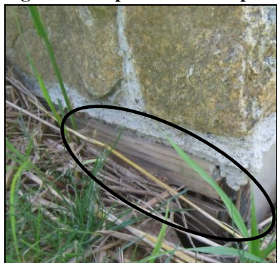
Figure 20 Wood forms left under stone and in contact with soil(siding & retaining walls)
