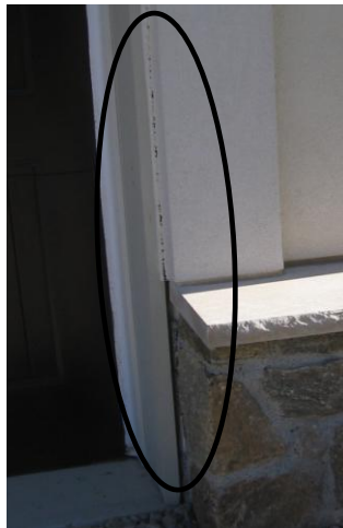
Figure 46 Examples of gaps around house, trim, railings and stone
