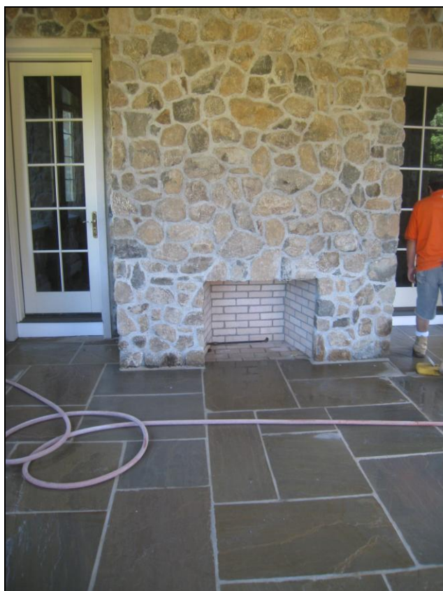
Figure 8 Slate/mortar repairs being made.
