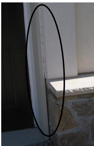
Figure 19 Examples of gaps around house, trim, railings and stone
