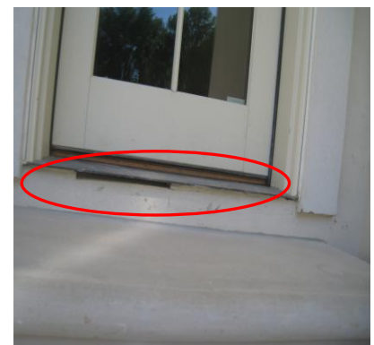
Figure 16 Gaps in caulking/mortar and ant hills. Gaps under rear door.
