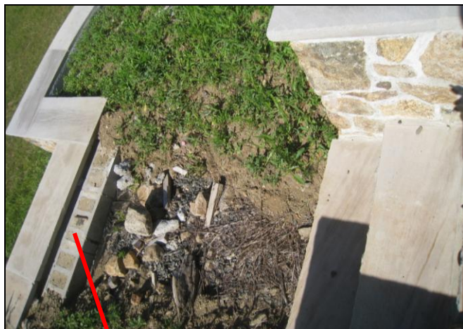
Figure 28 A & B Missing walk between retaining walls; fall hazard.
