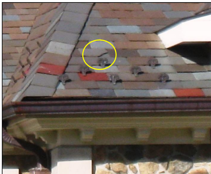
Figure 38 A & B Example of broken slate shingles
