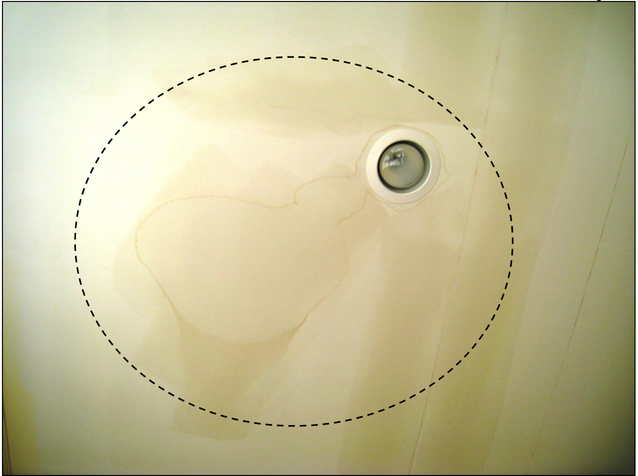
Figure 25 Water stains; indication of leaking above. See roofing section.
