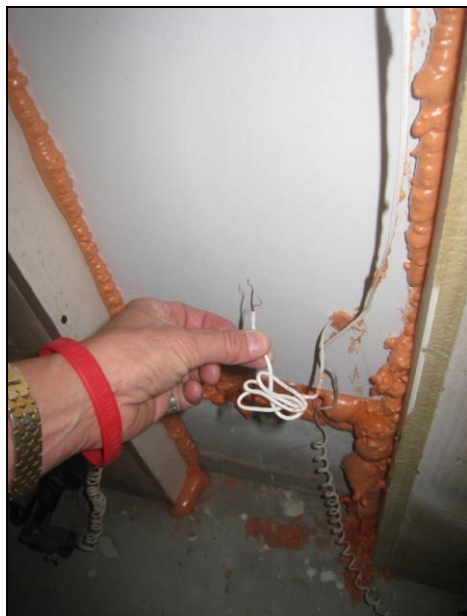
Figure 23 Loose wires by garage doors; further evaluate. Expansion foam everywhere; not recommended.
