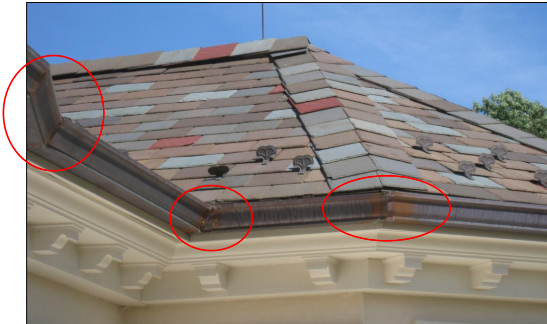
Figure 15 A, B, C & D Indication of leaking gutters and spillage marks. Ruts in soil below.
