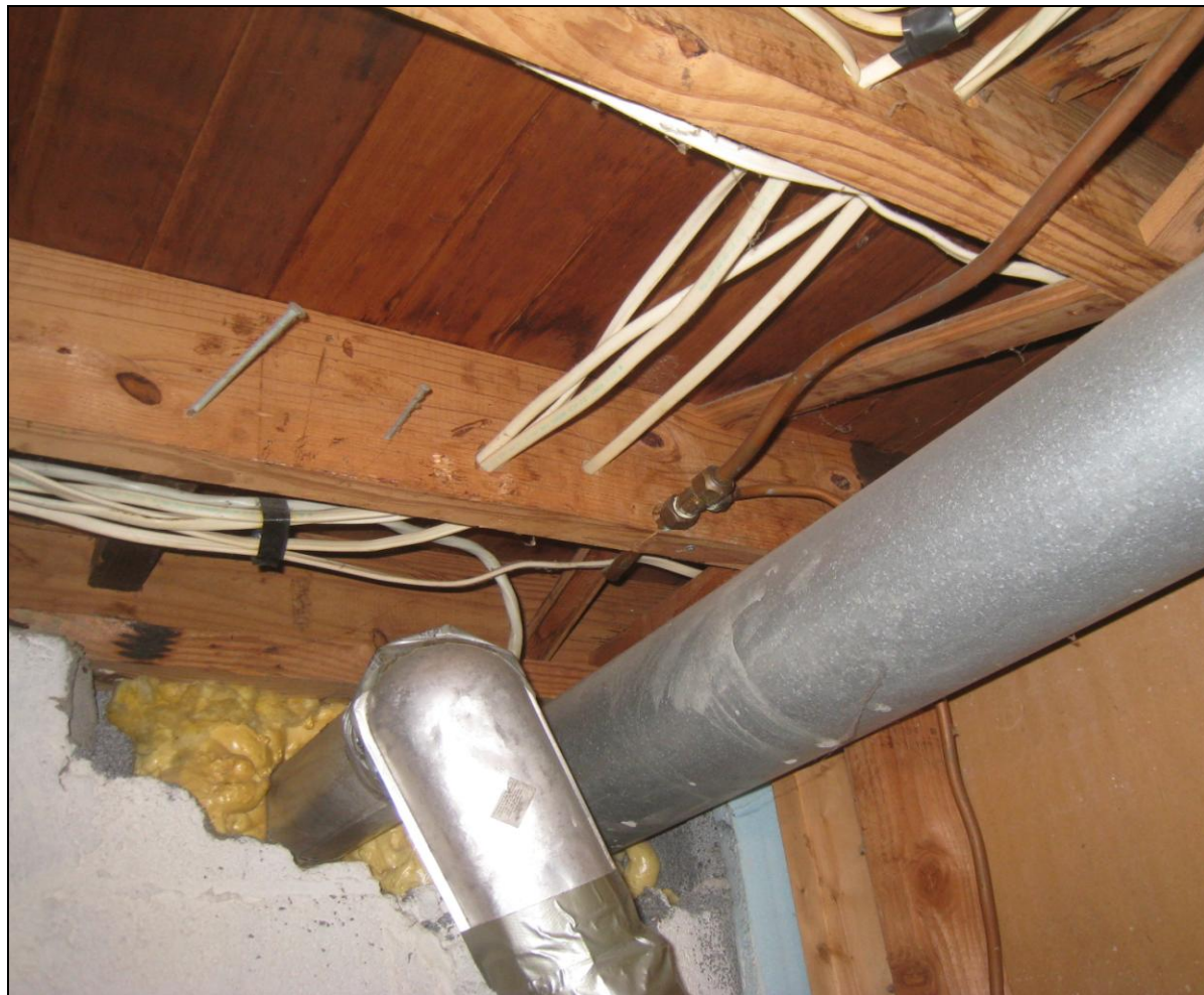
Figure 9 Damaged concrete wall where vented installed; have structure evaluated. Expansion foam is not recommended as a seal or repair.
