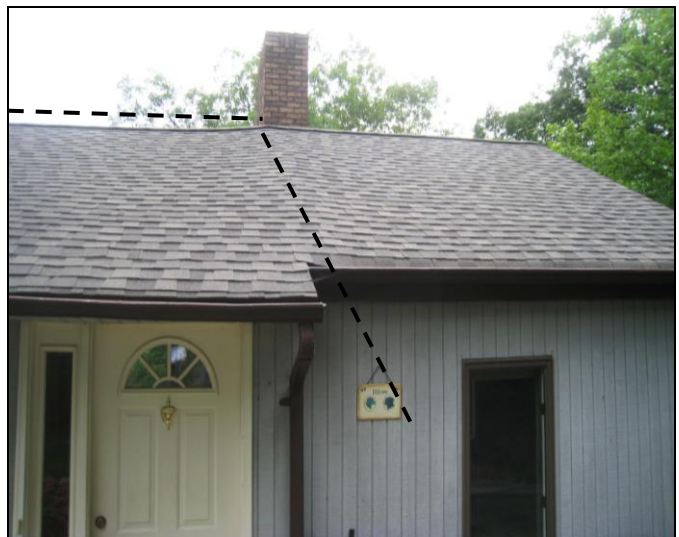
Figure 6 Right side addition; difference in roofline/dip. Obtain all township permits.
