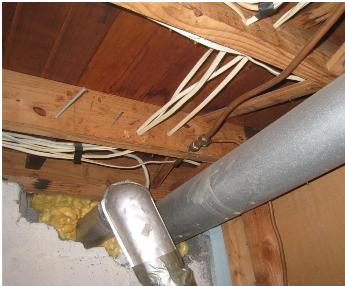
Figure 18 Damaged concrete wall where vented installed; have structure evaluated. Expansion foam is not recommended as a seal or repair.
