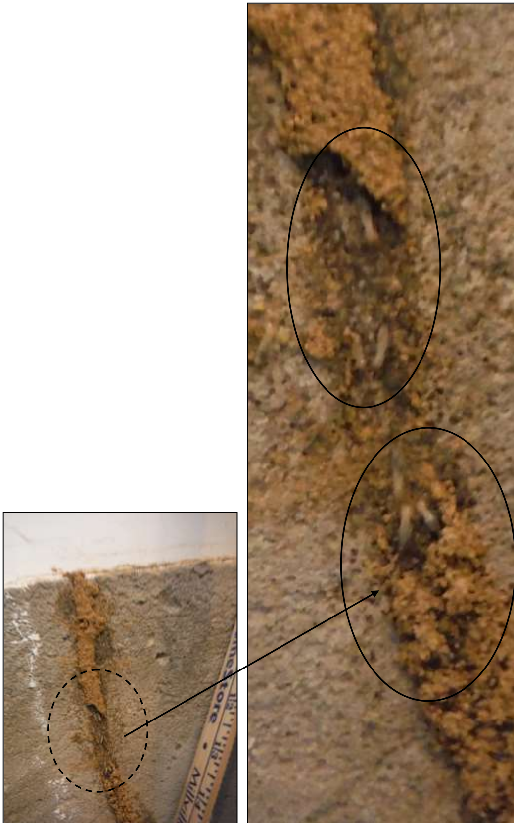
Figure 3 Live termite inside shelter tubes; scattered when tubes broken open and light hit them.
