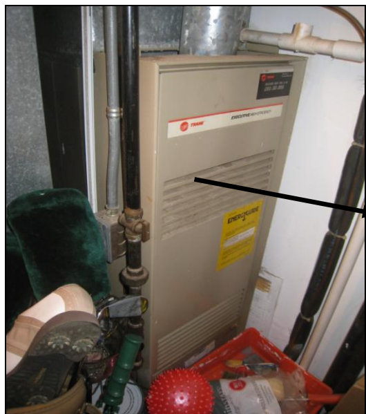
Figure 14 A & B Clutter poses a fire hazard in utility room. Heavy corrosion inside furnace; have evaluated now.
