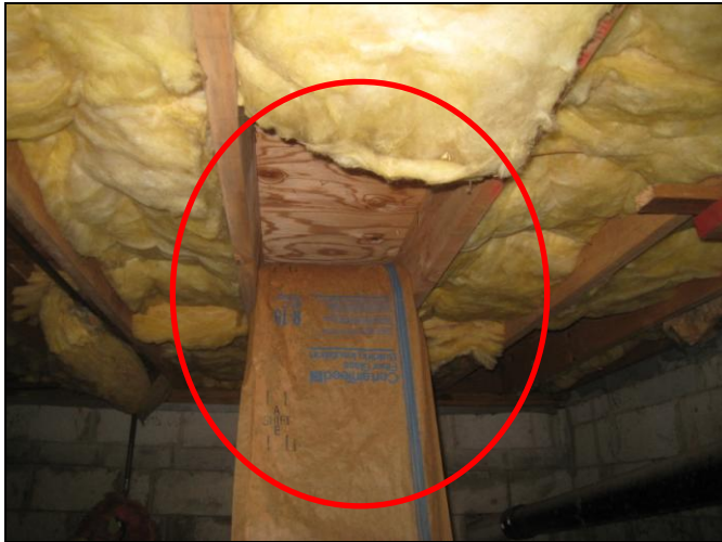
Figure 9 A & B Loose hanging insulation in crawl space.
